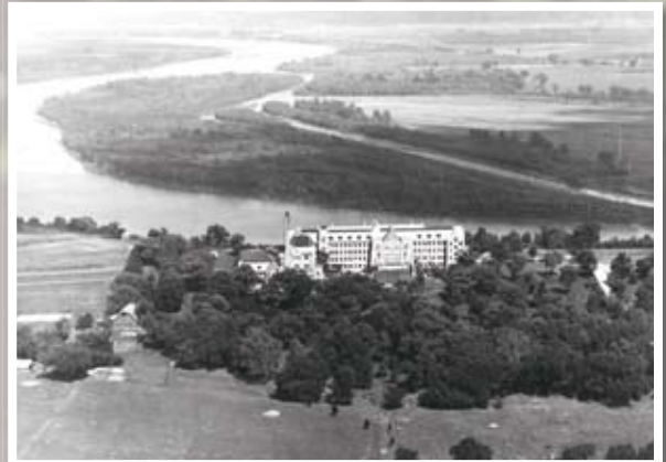
AERIAL VIEW OF THE ABBEY & MISSOURI RIVER VALLEY
