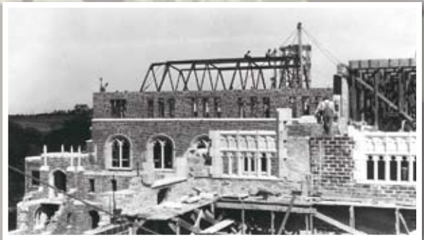
ST. BENEDICT’S ABBEY DURING CONSTRUCTION, 1927-29 (Incidentally, famed aviator Amelia Earhart’s birthplace is located just blocks from the abbey. As construction began on the new Gothic abbey in 1927, Ms. Earhart was about to be named the first female officer of the National Aeronautical Association.)
